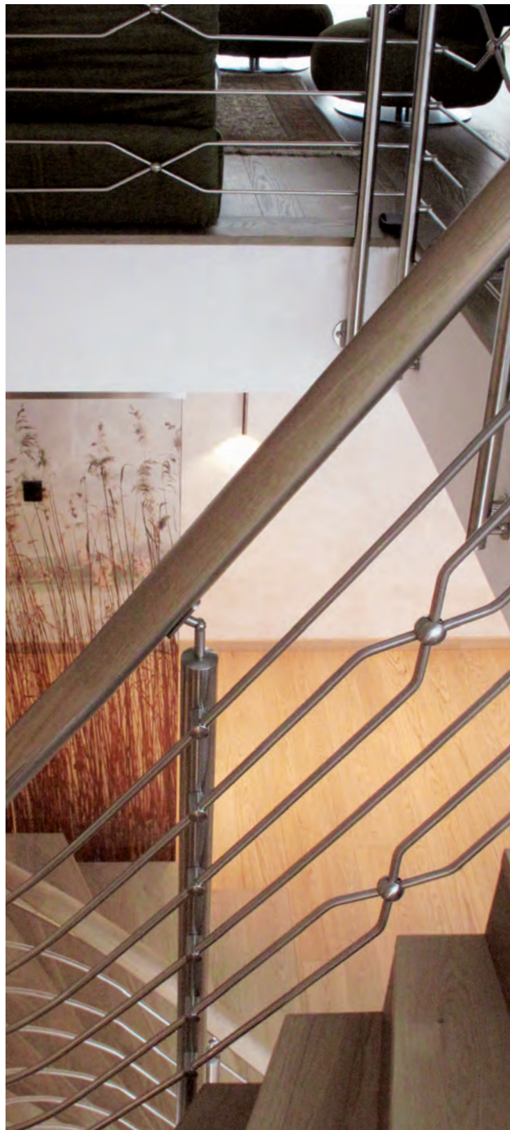
Sfere vuote con foro filettato, satinato Hollow spheres, with threaded inserts, satin finish
